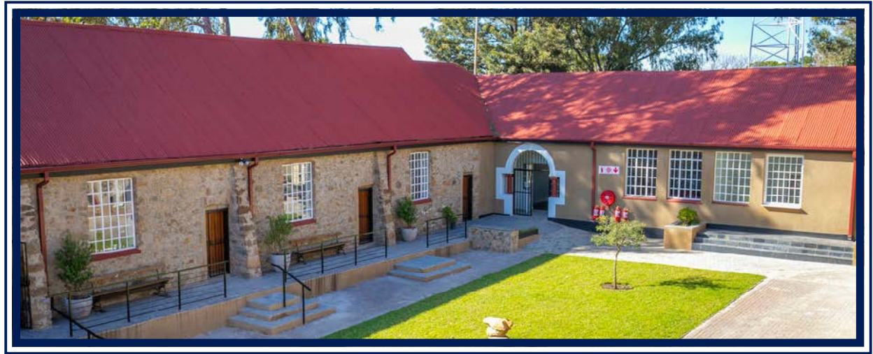
A Renovated and Restored St David's Marist Inanda Alex Campus 2023
